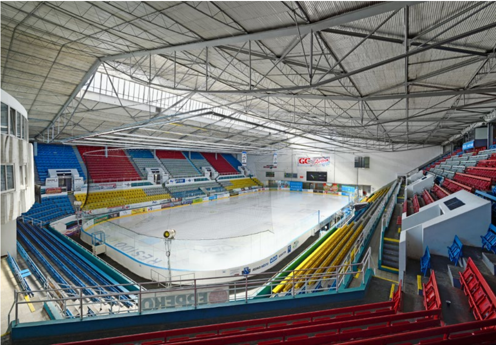
Fig. 3. Multipurpose hall (now Gascontrol Arena), view of the sports surface, tribunes and roof structure, Havířov-Podlesí, 1965–1968, photo: Roman Polášek, 2019
