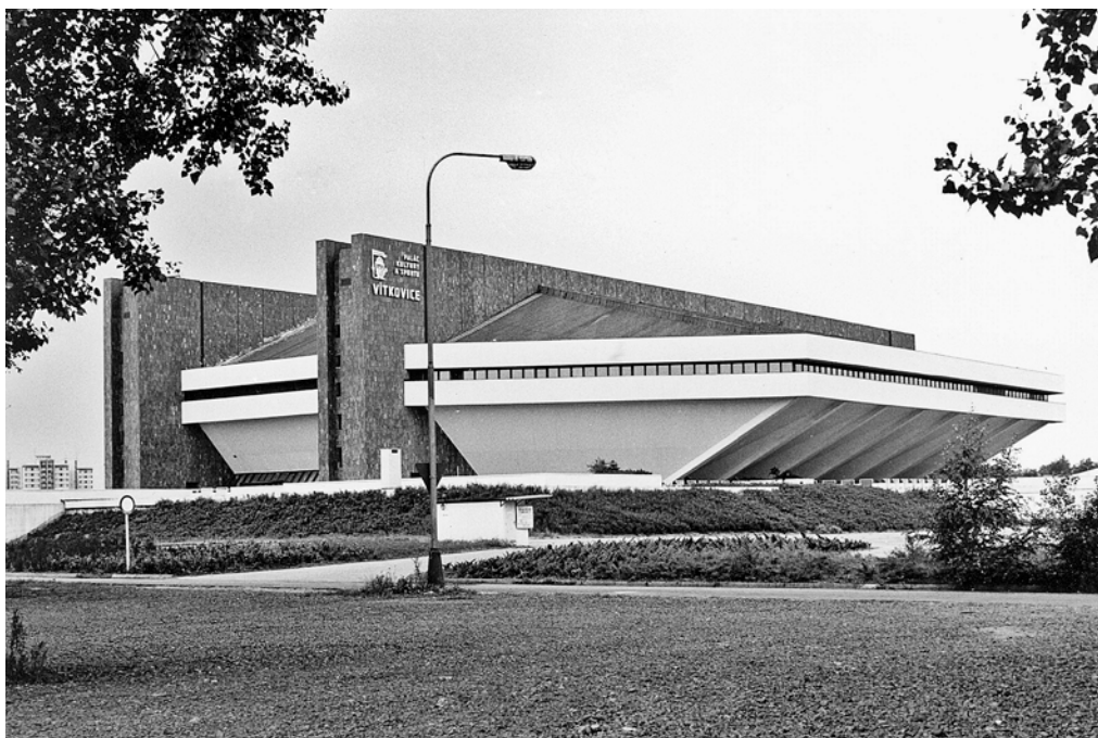
Fig. 11a. Palace of Culture and Sport (now Ostravar Arena), view from the southeast, Ostrava-Zábřeh, 1976–1986, Vladimír Dedeček, Stavoprojekt Bratislava, photo: unknown author, circa 1986, source: archive of the Institute of Construction and Architecture of the Slovak Academy of Sciences
