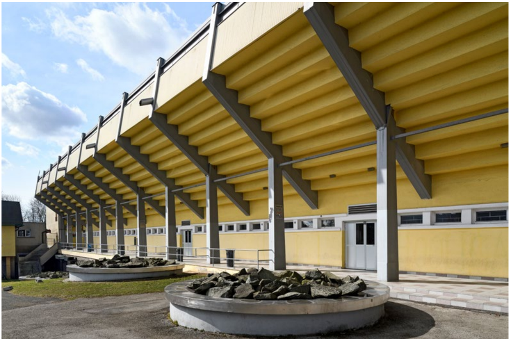
Fig. 2. Multipurpose hall (now Gascontrol Arena), eastern side façade with gargoyles and areas for collecting rainwater from the hall roof, Havířov-Podlesí, 1965–1968, Josef Hrejsemnou, Stavoprojekt Ostrava, photo: Roman Polášek, 2019
