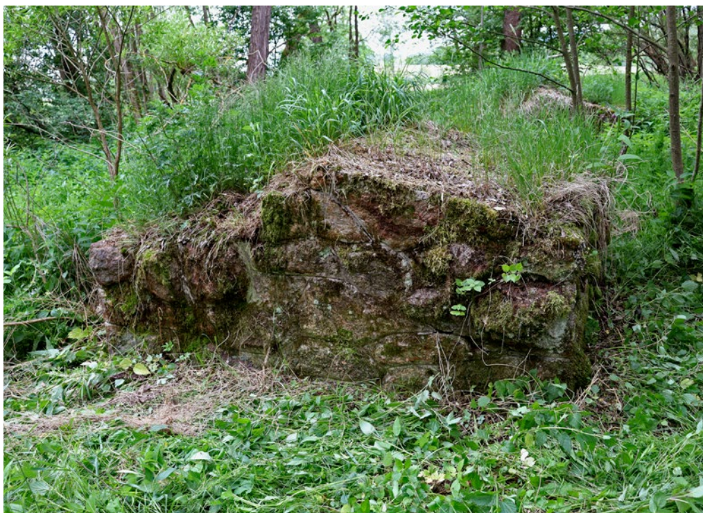
Fig. 2. Blansko near Kaplice, the Ponholz barrier, the side of an uncovered land pier, with the fifth pier behind, photo: the author, 2024
