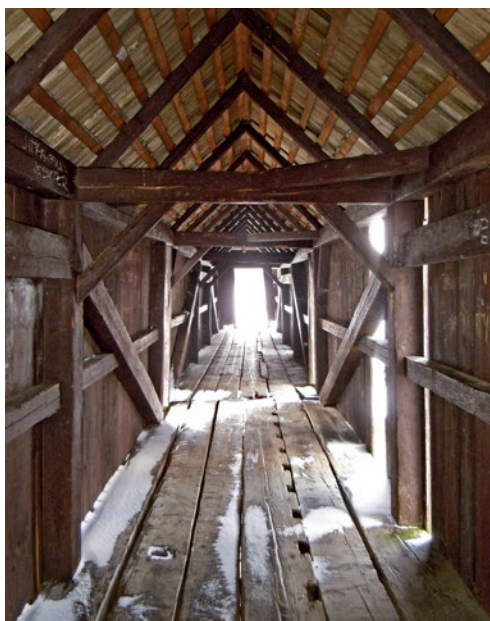
Fig. 21. Lenora, the Vogelberg barrier interior, state before the last repair (2012–2013), the beams were repositioned during previous repairs (e.g. in 1985), the beam with mortises has been dated to the 1860s by dendrochronology, photo: Radek Liška, 2012
