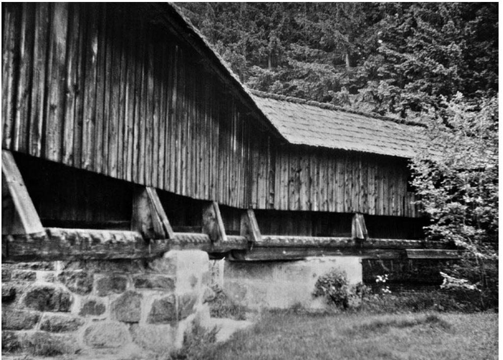
Fig. 6. Blansko near Kaplice, the Ponholz barrier, the front view reveals the mortises in the beam against which the bar screen bars were propped, photo: V. Šolc, 1955, source: Etnologický ústav AV ČR, v.v.i., photo documentation collection Prague, sign. 5958 HK
