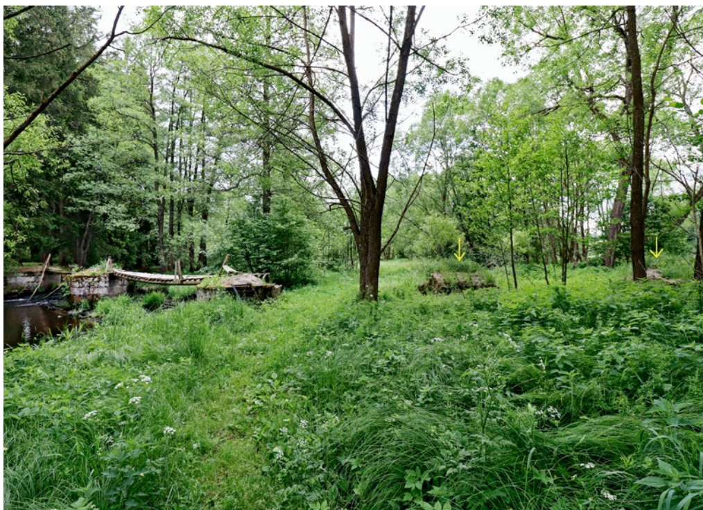
Fig. 1. Blansko near Kaplice, the Ponholz barrier, general view upstream the River Černá, marking the land piers, photo: Marie Hansová, 2024
