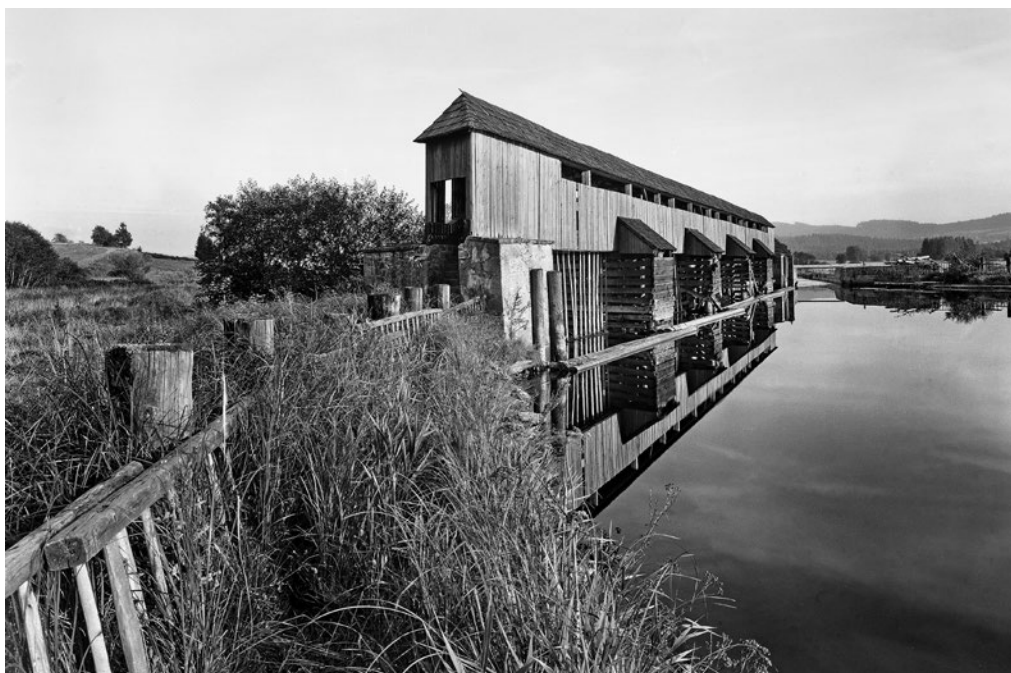
Fig. 17. The Spitzenberg (Hory) barrier on the Vltava near Želnavá, photo: Vladimír Hyhlík a Věra Pospíšilová, 1953, source: NPÚ Photo Archives, GnŘ, collection of photographic documentation
